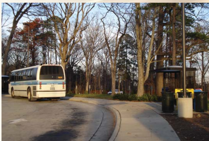
A park-and-ride lot in rural Chatham County, NC provides easy accessibility to free public transportation serving the Town of Chapel Hill and the University of North Carolina-Chapel Hill.
