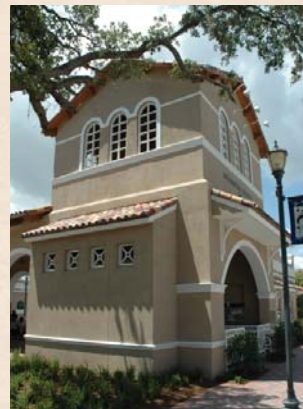
Fort Pierce "Green" Intermodal Transfer facility.
