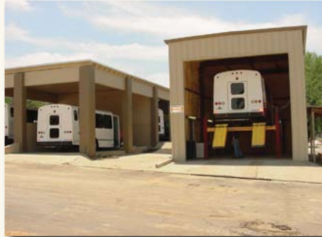
New bus inspection and water testing bays
